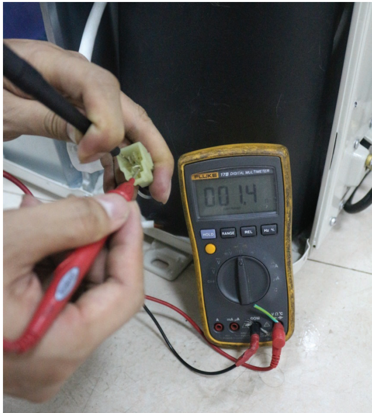
Fig. 64 – Test the resistance of the windings
