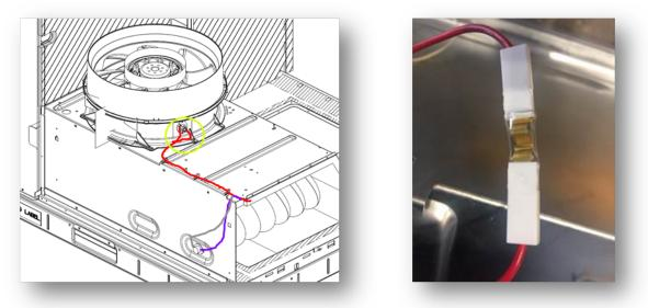
2. Remove the manual reset fan limit switch from the stator, and install the new automatic reset limit.
